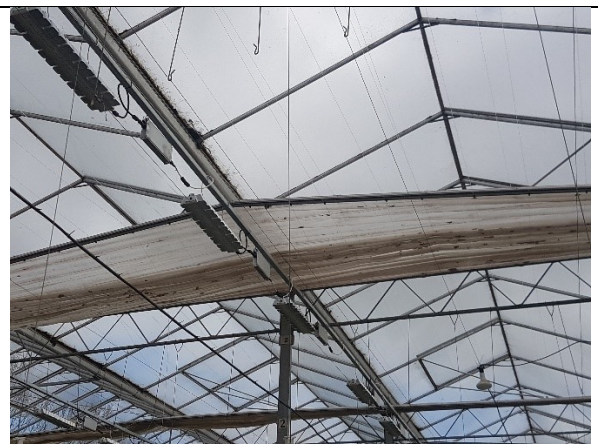
Figure 4 Lights in place, with insulation curtains behind. These curtains will be replaced with blackout blinds in August.
